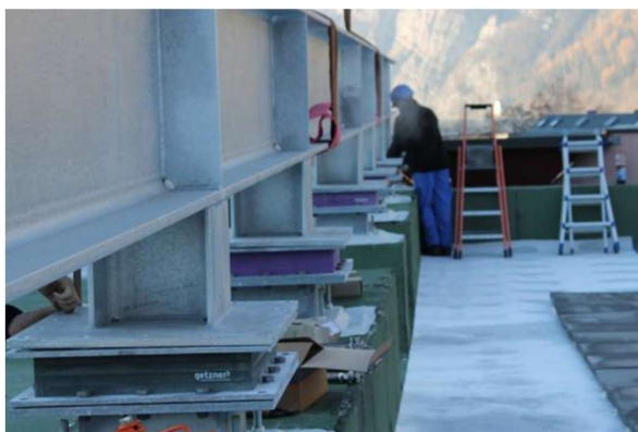
Figure 6 HRB HS Sylodyn Elastomeric Pad
