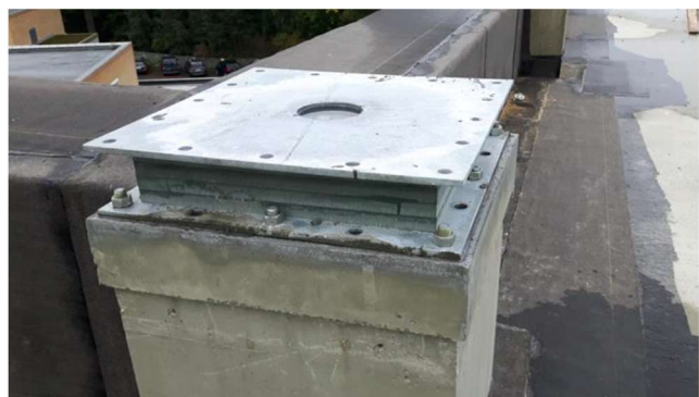
Figure 7 HRB HS Sylodyn Elastomeric Pad
